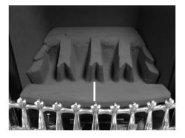
c) Fit five of the large sized coals onto the front ceramic rail, ensuring that they are evenly spaced. Use the recess's in the front ceramic rail as a guide for placement. (See fig. 3 below)
